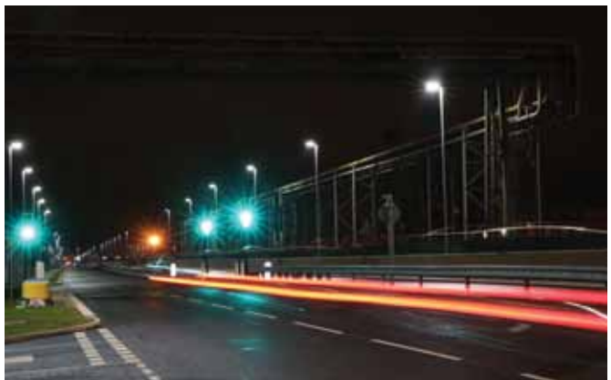
As part of redevelopment work at the Llanwern Steel Works, a new link road connecting a newly built housing estate was created. Lucy Zodion supplied products for the street lighting infrastructure for this link road.
